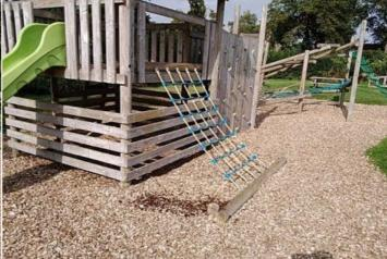
**Finding:** The net anchor forms a hard object within the impact area of the equipment in contravention of the requirements of BS EN 1176 Part 1
