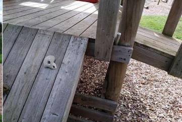
**Finding:** There is/are finger entrapment/s in the frame and the item fails to meet the requirements of BS EN 1176 Part 1
