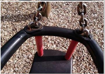
Finding: There is surface corrosion present on the fixings
