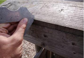
**Finding:** The item has exposed edges and corners with a **Action:** Provide a 3mm radius to all exposed edges and radius of less than 3mm and fails the requirements of BS EN corners 1176
