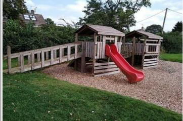
**Finding:** The height of the slide runout is in excess of 200mm and fails the requirements of BS EN 1176 Part 3
