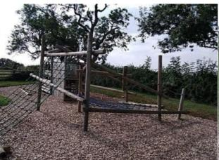
**Finding:** The net anchor forms a hard object within the impact area of the equipment in contravention of the requirements of BS EN 1176 Part 1
