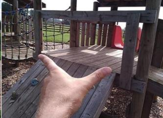
**Finding:** The platform provides access to a steep play element via a barrier with a width exceeding 1200mm and this fails to meet the requirements of BS EN1176 Part 1.
