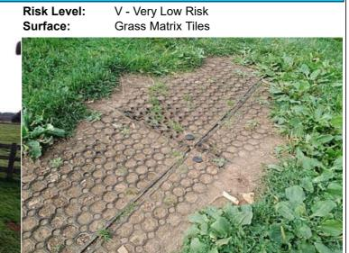
**Finding:** Fixing Pins have been installed in the impact areas **Action:** Remove pins from impact areas of the grass mats
