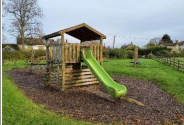
Finding: The safety surface is low and the membrane is exposed creating trip points
