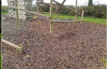
Finding: The depth of the loose fill surfacing is lower than the recommended depth specified in BS EN 1176 for a fall height over 2.0m. A minimum depth of 400mm is recommended (including an extra 100mm to allow for compaction and displacement as per BS EN 1176 Part 1 -Table 4)
