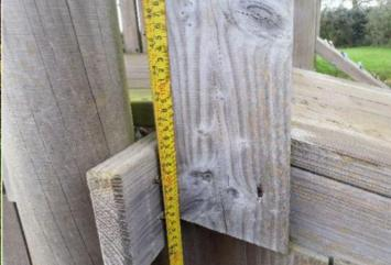
**Finding:** The unit is easily accessible and should have the appropriate barriers installed to meet the requirements of BS EN 1176 Part 1 as the height of the unit exceeds 600mm
