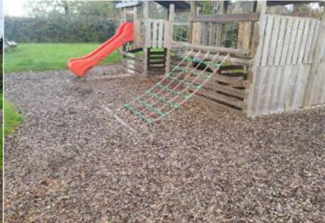
Action: Top up loose fill surfacing to recommended levels
