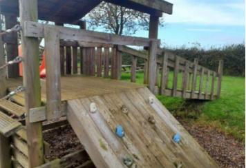
Finding: The unit is easily accessible and has an opening in Action: Monitor - No remedial work recommended the barrier to steep play elements in excess of 500mm in contravention of BS EN 1176 Part 1
