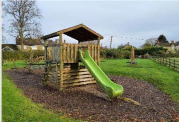
**Finding:** The depth of the loose fill surfacing is lower than the recommended depth specified in BS EN 1176 for a fall height over 2.0m. A minimum depth of 400mm is recommended (including an extra 100mm to allow for compaction and displacement as per BS EN 1176 Part 1 - Table 4)
