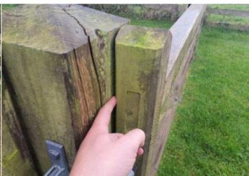
**Action:** Provide a 12mm gap throughout full range of motion at both sides of gate
