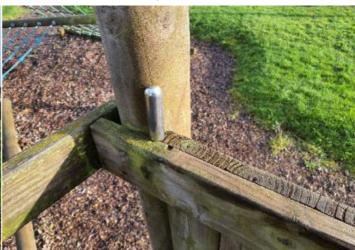
**Finding:** There is/are finger entrapment/s in the barriers and **Action:** Monitor - No remedial work recommended the item fails to meet the requirements of BS EN 1176 Part 1 4.2.7.6 Entrapment of fingers
