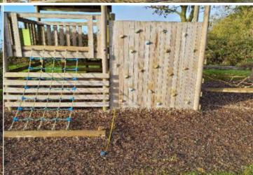
**Finding:** The rope net anchor beam forms a hard object within the falling space of the equipment in contravention of the net the requirements of BS EN 1176 Part 1
