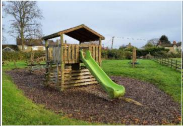
**Finding:** There are openings leading from platforms in excess of 1.0m in height to steep play elements and no hand supports complying with grip or grasp are provided, in contravention of BS EN 1176 Part 1: 4.2.9.4
