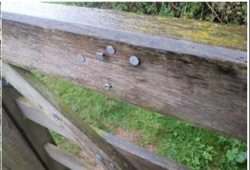
Finding: There are projecting nail ends and staples present Action: Remove and provide more appropriate fixings if
