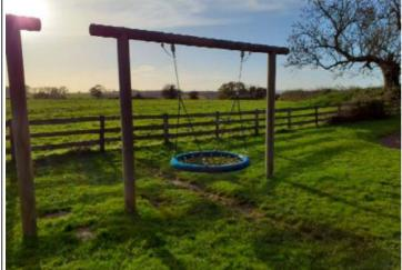
**Finding:** BS EN 1176 requires an additional 0.5m of unobstructed space at each end of the swing surfacing area. This is a relatively low risk finding and no remedial action is recommended at this point.
