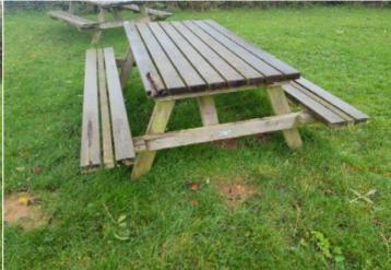
**Finding:** The table/s is/are not secured to the ground and there is some potential for the item/s to be moved within falling spaces of equipment
