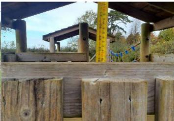
Finding: The height of the barrier(s) is insufficient and fails Action: Monitor - No remedial work recommended to meet the requirements of BS EN 1176 Part 1
