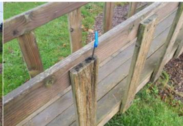
Finding: There are areas or parts of the timber barriers on Action: Replace all affected timbers the structure that have rotted
