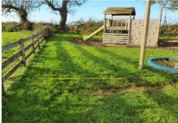
**Finding:** The surfacing dimensions are short and do not meet with the requirements of the current applicable standard
