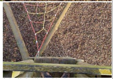
**Finding:** There are falls in excess of 600mm between adjacent components on the structure, in contravention of the recommendations set out in BS EN 1176 Part 1; 4.2.8.4
