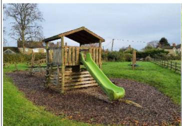
**Finding:** There is/are finger entrapment/s in the guardrail and the item fails to meet the requirements of BS EN 1176 Part 1 4.2.7.6 Entrapment of fingers
