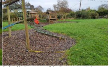
**Finding:** The surfacing dimensions are short and do not meet with the requirements of the current applicable standard
