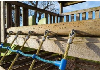
**Finding:** There is/are finger entrapment/s in the rope net framework and the item fails to meet the requirements of BS EN 1176 Part 1 4.2.7.6 Entrapment of fingers
