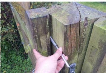
**Action:** Provide a 12mm gap throughout full range of motion at both sides of gate
